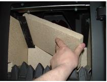
Lift the Baffle Brick and slide to the left. When the right side of the Brick clears the Baffle Support, lower the Brick into the Fire Box and remove.
