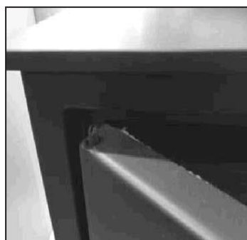
Upper door pin attached to door
