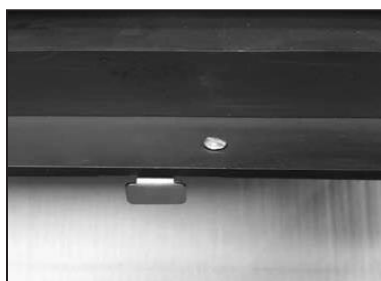
Upper door pin attached to door
