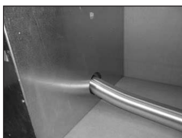
Ø63mm flexible pipe pushed through outer box
