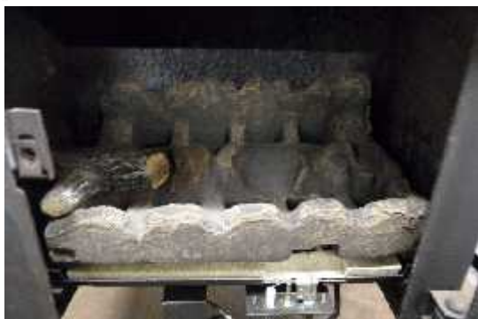
Photo 6: Installing Log A.
