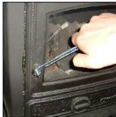
Photo 2: Removing door fixing bolt
