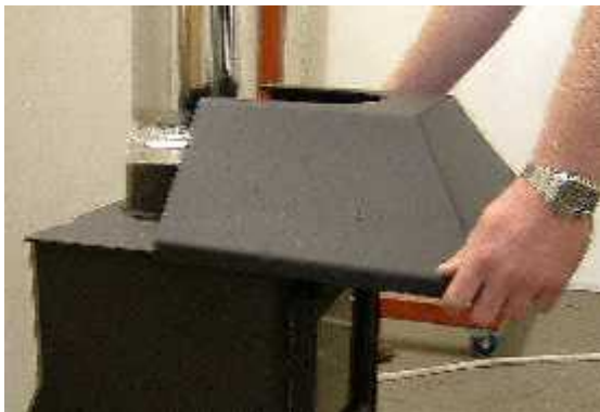
Photo 11: Fitting a canopy
