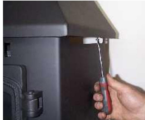
Photo12: Securing the canopy.
